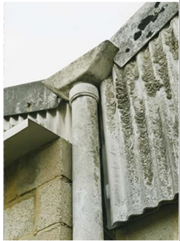
Asbestos cement downpipe, hopper and profile sheet
